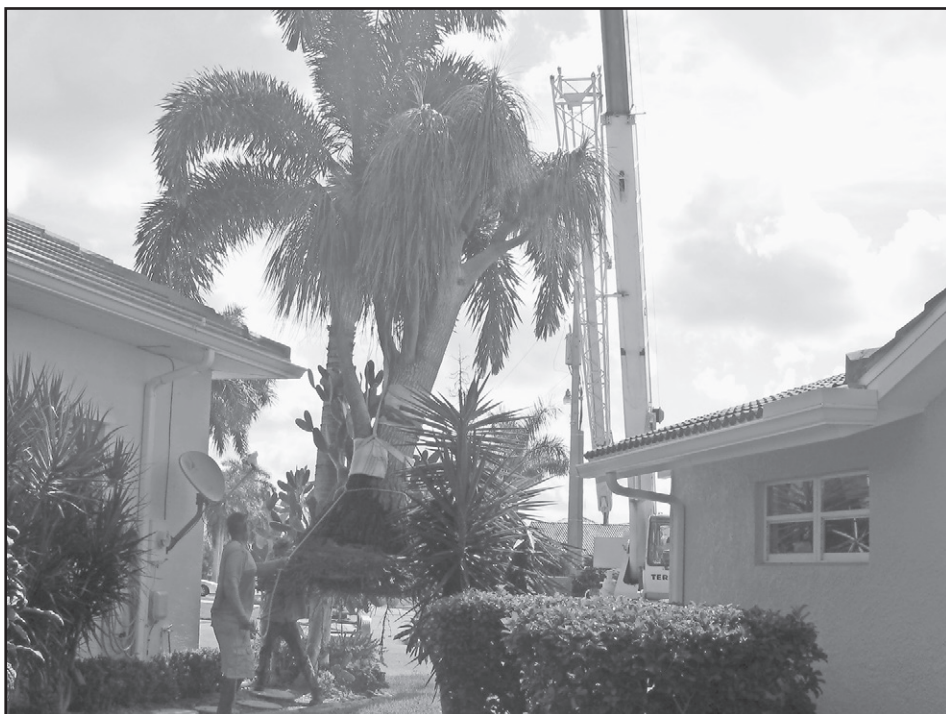
Danny Jones keeps a grip on the guide rope as crane operator Scott Graber walks the tree down the driveway.
